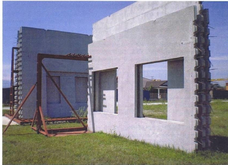
Fig. 2 Panels of HC precast wall system
