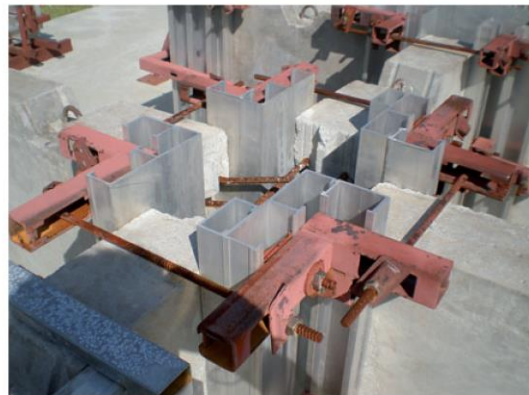
Fig. 3: Example of '4' shaped modular mould and installation
