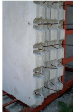
Fig. 4: Double groove lines for waterproofing
